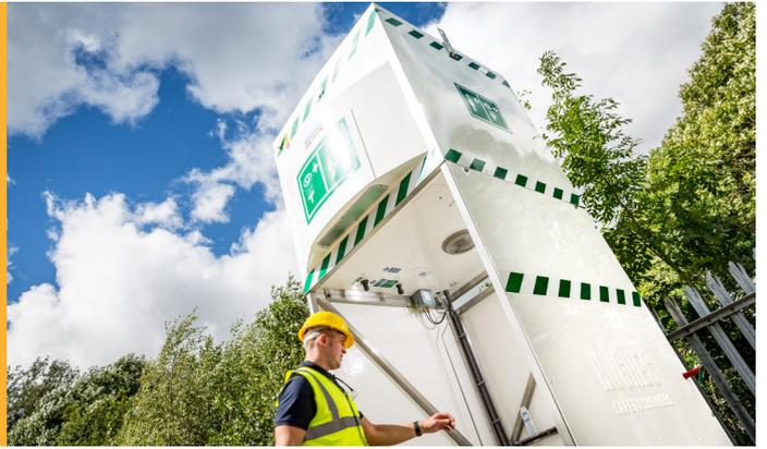
Emergency safety showers and eye wash stations are essential for sites where workers could come into contact with hazardous chemicals. In some environments providing this life saving equipment can be challenging, for instance a consistent supply of potable water cannot be guaranteed, or a tepid temperature can be difficult to maintain due to extreme ambient temperatures.
