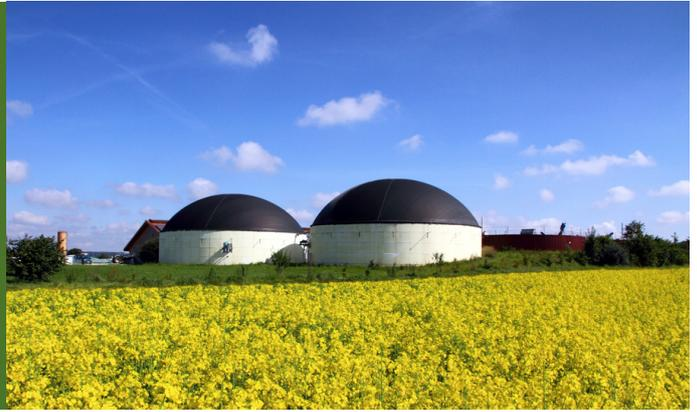
**Anaerobic digestion is a collection of processes which naturally breakdown organic matter to eventually produce biogas - a methane rich gas which is burned to produce both heat and electricity. The methane can also be used as vehicle fuel or injected into the gas grid. The industry is growing fast and is forecast to continue to do so with many farmers adding bio-gas plants alongside their everyday farming activities.**
